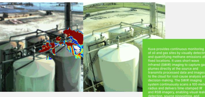
of oil and gas sites by visually detecting infrared (SWIR) imaging to capture gas transmits processed data and images to the cloud for root-cause analysis and decision-making. The SWIR imaging system continuously scans a 100-meter radius and delivers time-stamped IR and RGB imagery, enabling visual leak detection, source pinpointing, and rapid root cause analysis.
